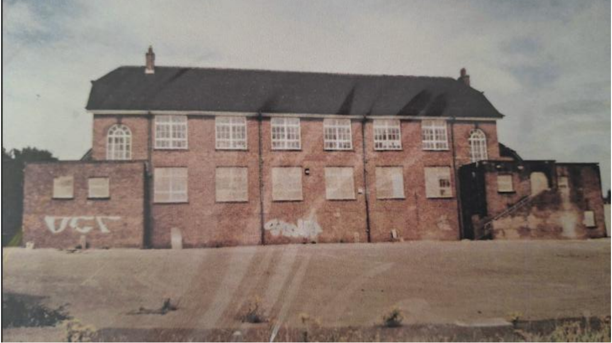
This is the rear of the school after it was boarded up.
